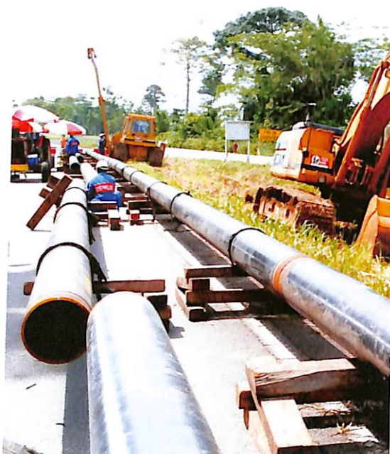
The country participates in the West African Pipeline Company
