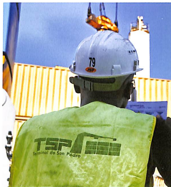
A terminal for refined fuel is being built at the Port of San Pédro
