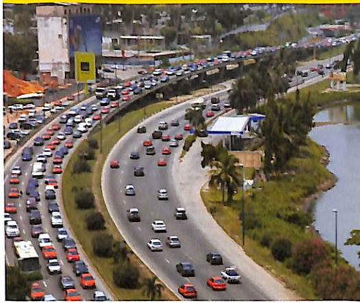
The road system is one of the largest and densest in West Africa
